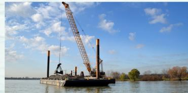
**RESTORATION:** Reefs are built with marine construction vessels that place quarried limestone rock on the river bottom.
