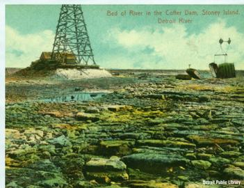
Sections of the Detroit River were drained and blasted to create deeper shipping channels, which damaged important fish habitat. These historical photos show the river bottom before (left) and after (right) excavation of the Livingstone Channel, around 1910.
