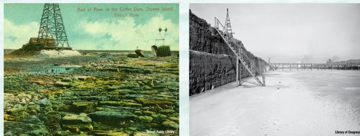
Sections of the Detroit River were drained and blasted to create deeper shipping channels, which damaged important fish habitat. These historical photos show the river bottom before (left) and after (right) excavation of the Livingstone Channel, around 1910.
